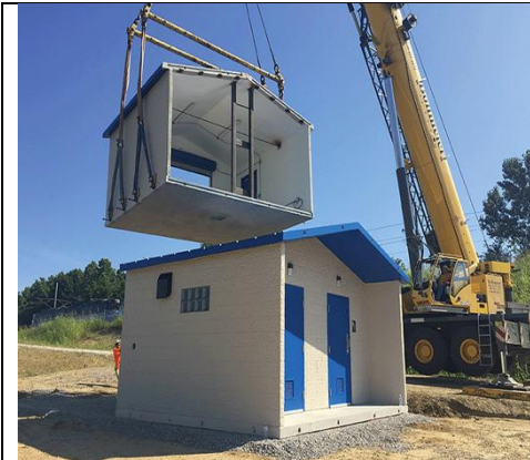
Figure.1 preparing to put abuilding
