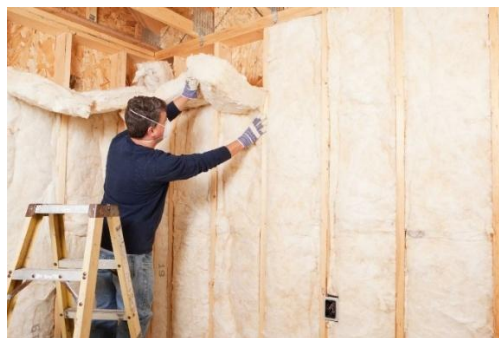
Figure 4. (An illustration of a man installing fiberglass insulation)
