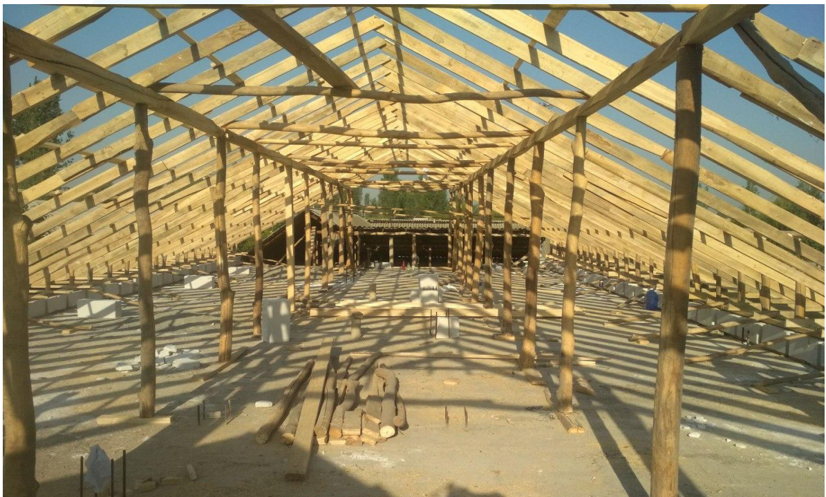
General view of wooden roofing elements .
